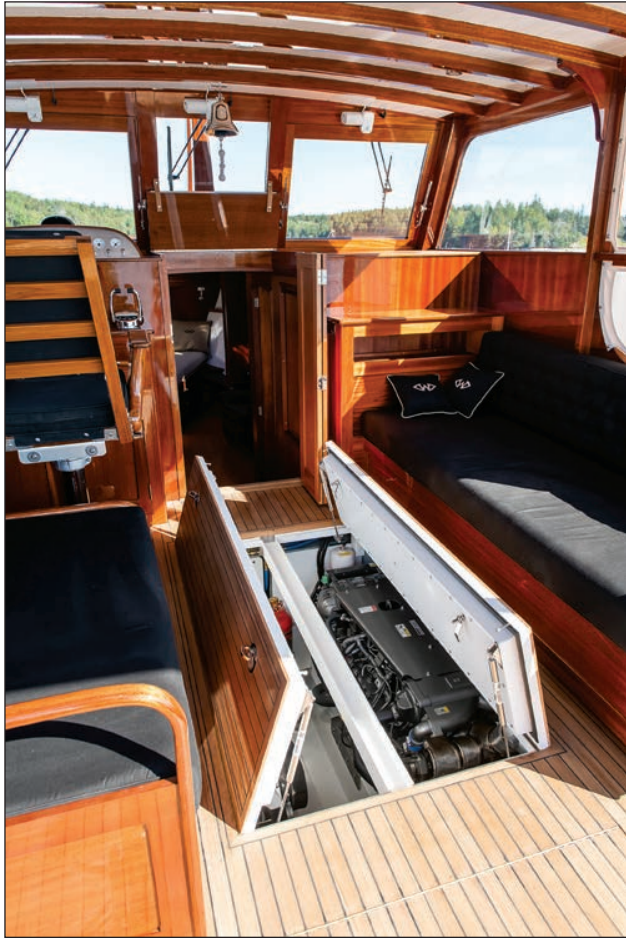
The two Yanmar diesel engines are installed in a compact engineroom below the cockpit sole but with additional service access through the bottoms of the side seats. The 13.5kW Cummins Onan genset is aft of the engines, and farther aft, where Hemingway would have had a large icebox for fish, LEGEND has a Seakeeper roll-dampening unit.
